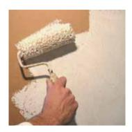
Apply one coat of PRIMER MINERAL that has been diluted 25% with water. It can be rolled, brushed or sprayed on; Let it dry 6 hours.
