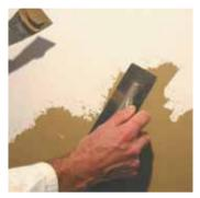
Apply first coat of MARMORINO with stainless steel trowel, skimmed in all directions, creating soft textured and organic designs. The grain of Primer Mineral must be covered; to avoid chatter marks work with a little bit more material with rounded motions, in all directions. Dry to "in love" or completely.
