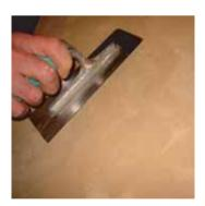
OPTION: when second layer is just set (before burnishing), use VEILCALCE TRANSPARENT light tinted or white and skim coat it over (non-diluted) with trowel, just to embed a very small amount of lime paint. You also can dilute VEILCALCE TRANSPARENT and brush it on, removing the excess with a trowel. Burnish when "in love" slightly to have an authentic mineral look.
