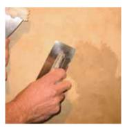
1 or 2 days later apply an optional coat of NEUTRAL or PEARLESCENT WAX using trowel or rag from wet to dry. Polish with "wooly" when dry after 1 or 2 hours. Note: waxing eliminates the mineral look of stone, but adds protection and depth.
