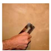
Apply second layer of MARMORINO with stainless trowel, when first coat is "in love" or completely dry. Work in diagonal passes from wet to dry; make sure everything is 100% covered and remove excess material (open the trowel angle slightly). Burnish lightly when still "in love".
