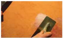
Both Options A & B: after 24 hours apply 1 coat of NEUTRAL or PEARLESCENT WAX with trowel, cheesecloth (always using small strokes from wet to dry) or a rag (circular motions).
