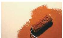
Apply first coat of tinted STUCCO TERRA with a roller (with a medium – heavy nap) to form peaks creating lots of texture.
