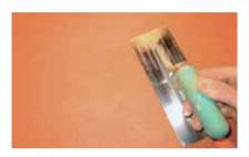
Option A (one step process): when product is just set ( before "in love" ), knock down the peaks with a stainless steel trowel working the same area in the same direction, then going to other areas in a different direction, to obtain stone effects.
