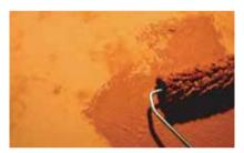
Option B (2 step process): after 48 hours, use the same roller and STUCCO TERRA (or different lighter color or shade), roll and skim right away (using both hands) in order to duplicate and accentuate the texture created in the first step.
