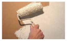
Apply one coat of PRIMER MULTI-USE rolled, brushed or sprayed. Let dry 6 hours.
