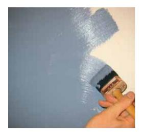
Apply the first coat of VEILCALCE (diluted 20%) with black bristle brush; work mixing circular and cross-hatch motions to create brush marks (or adjust your strokes to eliminate brush marks as much as possible). Let dry completely or "in love".
