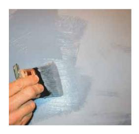
When dry or "in love", apply a second layer of VEILCALCE with the same dilution or from 20% to 30% with water; using same motions with the same brush; apply using diagonal strokes. It is possible to change the color or just a shade, however, lighter than 1st layer to create more contrast.
